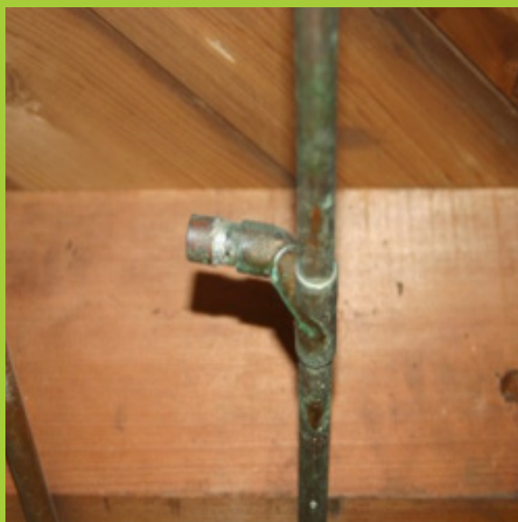
Photographs showing images of dead legs/ blind ends.
