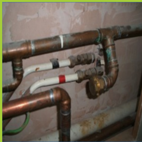
Photographs showing images of dead legs/ blind ends.
